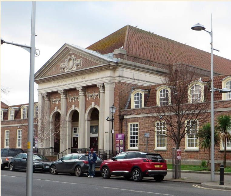
The Princes Theatre, within the Town Hall building, has little presence from the outside
