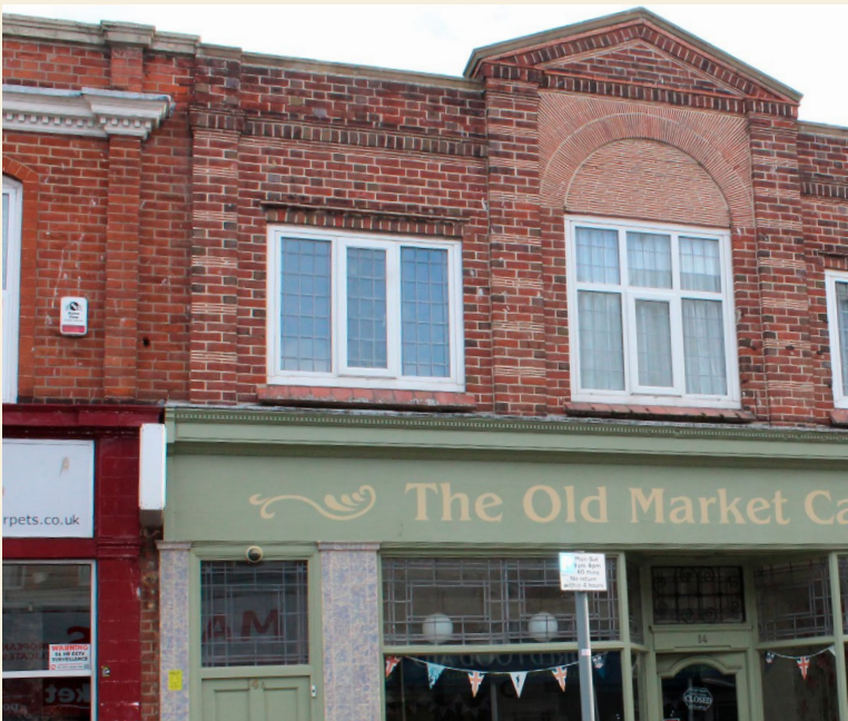
Much of the architectural character at upper levels goes unnoticed
