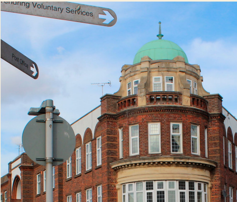
Corner buildings have architectural features that double as wayfinding in the town centre
